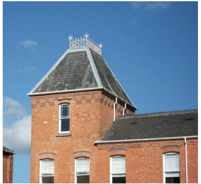
Above left: The architecture of the ward buildings includes slender sash windows with ashlar sills and arched brick lintels incorporating blue brick detailing. The roof is of Welsh slate with ridge tiles and the eaves are decorated with courses of projecting bricks. Above right: one of the four towers found on the ward buildings. These have pyramidal state roofs with wrought iron finials and brick eaves detailing.
