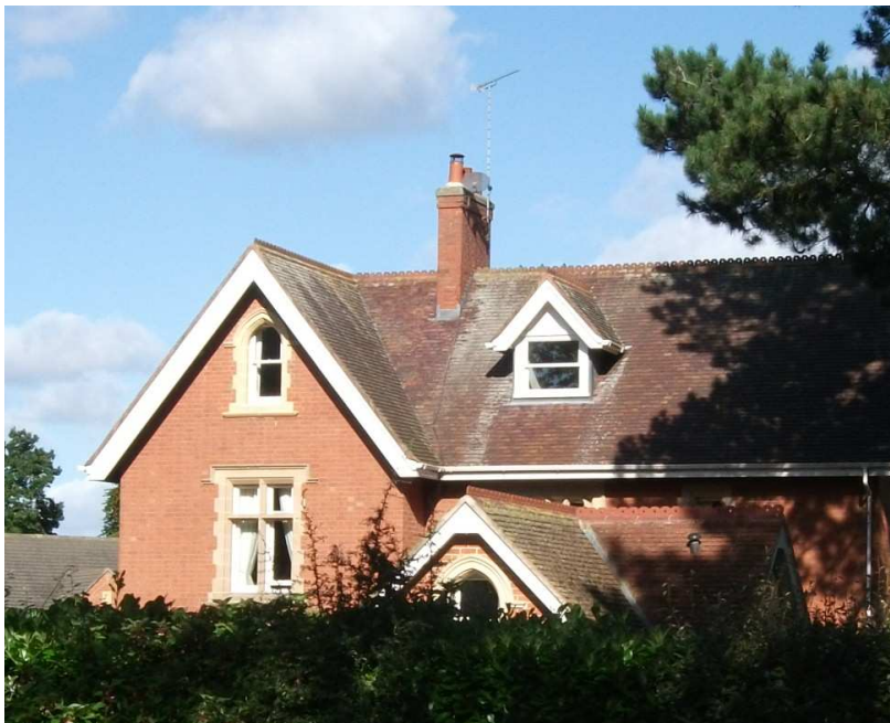
Above left: Professors House has an over sailing roof with timber barge-boards at the gables and ashlar mullioned and transomed sash windows. Above right: the administration building's central entrance was once the formal entrance to the hospital and is heavily decorated with ashlar detailing around the windows, door and clock face. The gable is further adorned with ashlar kneelers, parapet and finial and floral terracotta diaper work.
