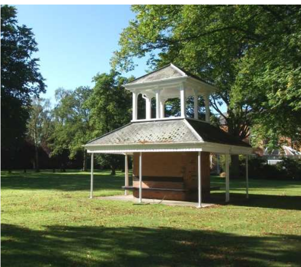
Above left: One of the four garden pavilions. These timber and cast iron structures were built around central brick ventilation shafts which provided fresh air to the hospital cellars through a network of underground tunnels beneath the grounds. Above right: late 20 th century detached houses on Berkeley Crescent.
