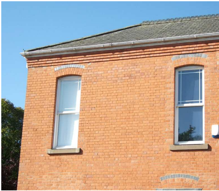
Above left: The architecture of the ward buildings includes slender sash windows with ashlar sills and arched brick lintels incorporating blue brick detailing. The roof is of Welsh slate with ridge tiles and the eaves are decorated with courses of projecting bricks. Above right: one of the four towers found on the ward buildings. These have pyramidal state roofs with wrought iron finials and brick eaves detailing.
