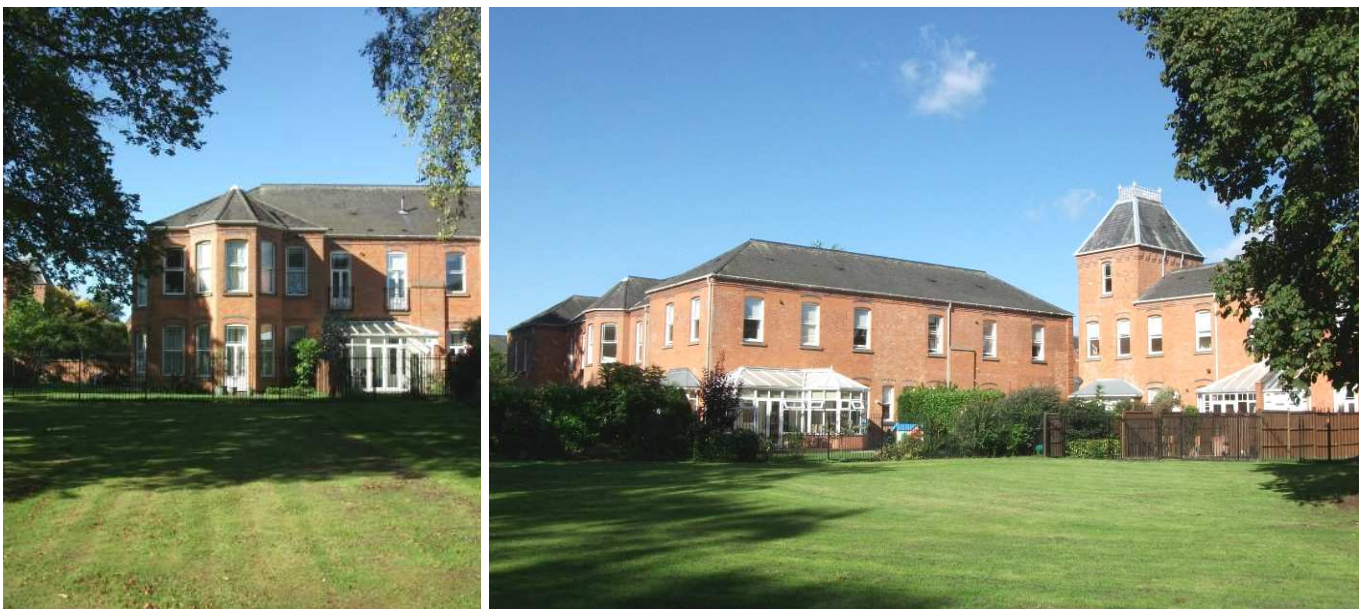
Above: The converted former ward buildings are of a typically restrained late Victorian character. Architectural detail and variety in the elevations is provided by full height bay windows and feature towers.
