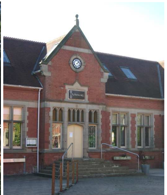
Above left: Professors House has an over sailing roof with timber barge-boards at the gables and ashlar mullioned and transomed sash windows. Above right: the administration building's central entrance was once the formal entrance to the hospital and is heavily decorated with ashlar detailing around the windows, door and clock face. The gable is further adorned with ashlar kneelers, parapet and finial and floral terracotta diaper work.
